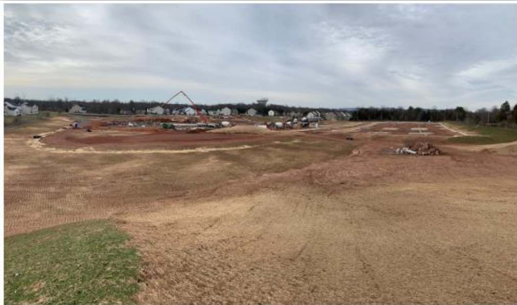
PANORAMIC VIEW OF SITE FROM NORTH EAST CORNER
