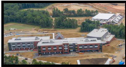
Paul VI HS - Loudoun Campus School Construction Underway (2019)
